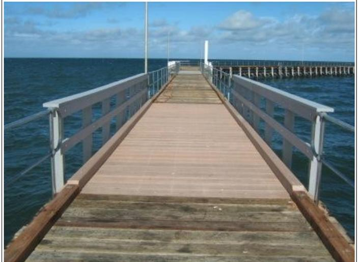
Image: Segment of Moonta Bay jetty repaired with recycled plastic.
